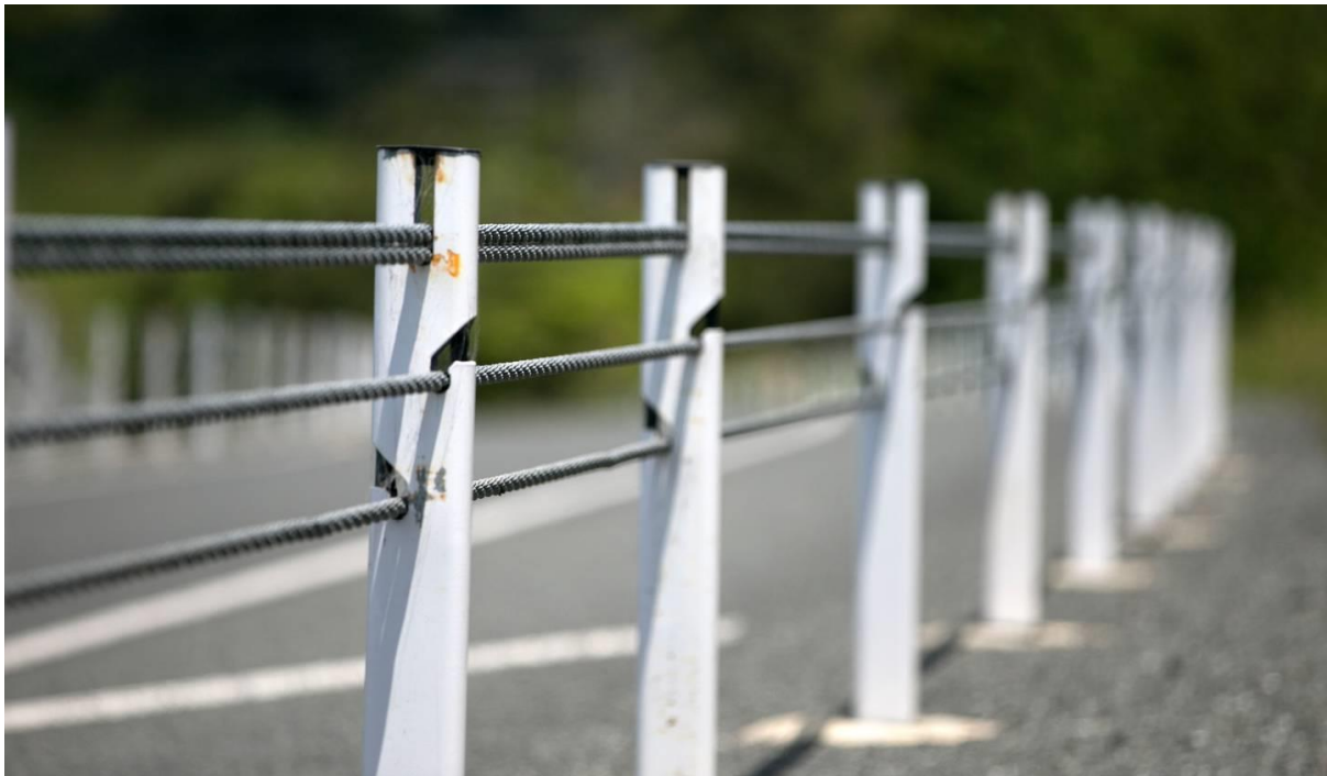
Flexible median barriers like this one have been put in on some stretches of Northland's state highways as part of Road to Zero. Photo / NZME
